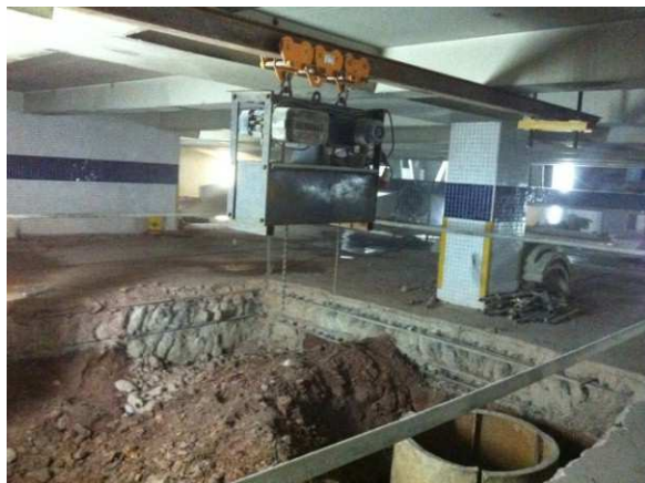
Setting-up of Caisson Frame
